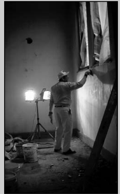
Plaster being repaired.
