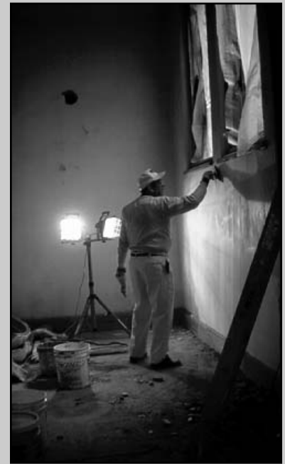
Plaster being repaired.
